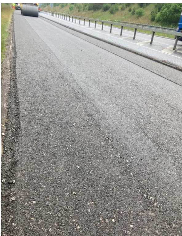
Fig. 2.7 (th): Overflade af BSM under tromling.
