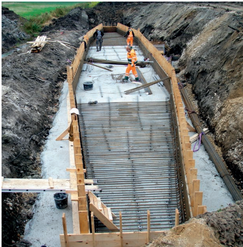
Form and reinforcement work on foundation for fauna passage
